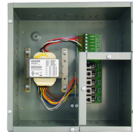
PSH200A-LVC Shown Without High Voltage Cover & Low Voltage Access Plate
